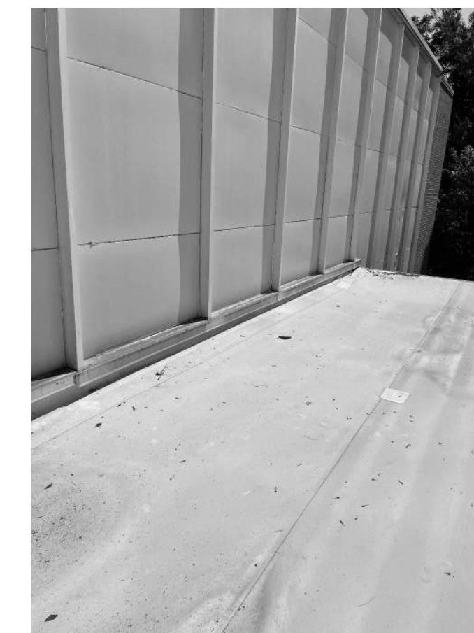
E.3 EXISTING FLASHING AT METAL PANEL. SEE NEW FLASHING DETAIL A1/A402.
