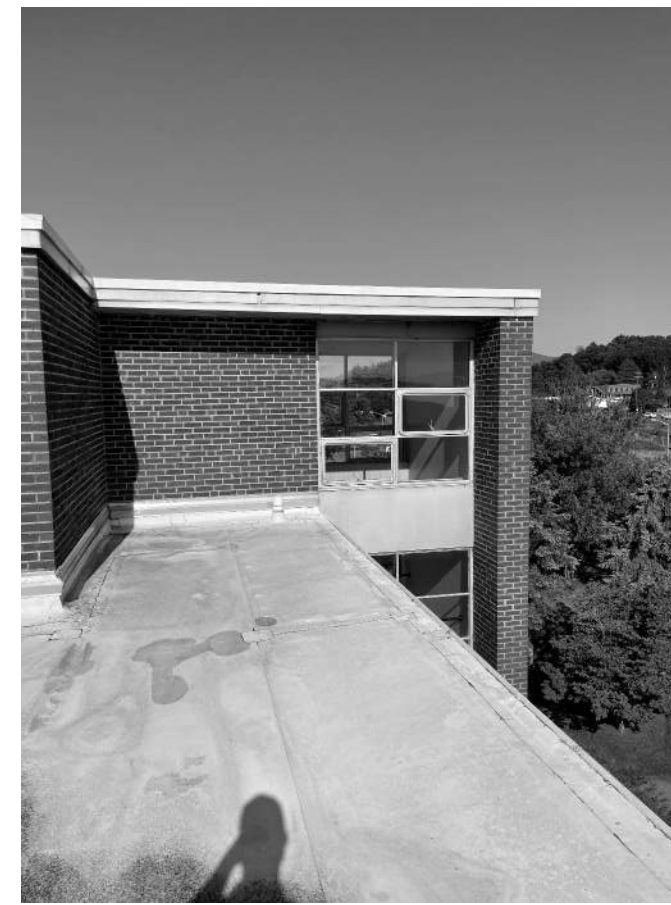
C.2 EXISTING MAIN STAIR.
