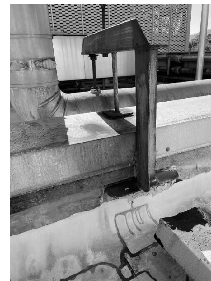
B.10 PIPING AND STAND TO BE REMOVED.
