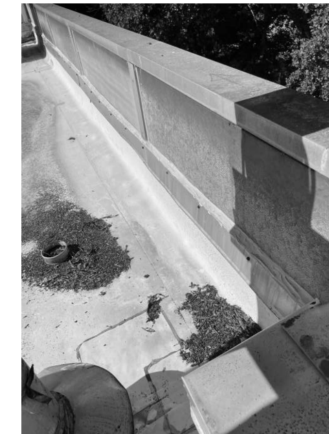
B.4 METAL PARAPET CONDITION. SEE C1/A402
