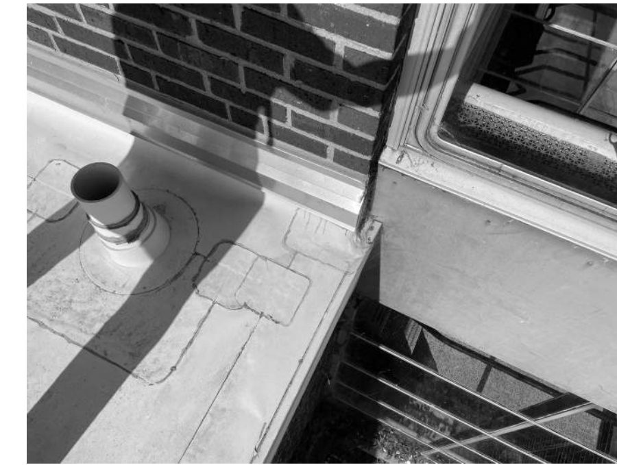
C.3 FLASHING AT EXISTING MAIN STAIR.
