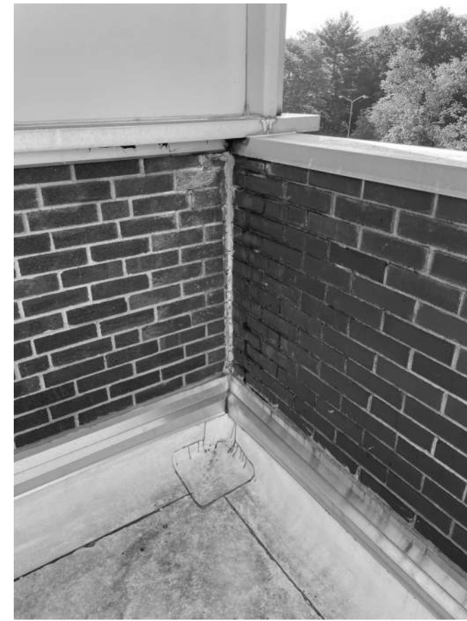
A.5 PARAPET TO BE REMOVED
